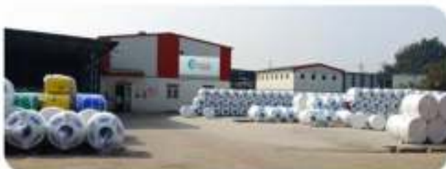
Manufacturing Plant - Sikandrabad (U.P.)
